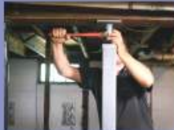
6. Fully tighten stabilizer.
