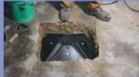
2. Place LightFoot into prepared space
