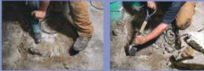
1. Prepare soil for footing placement
