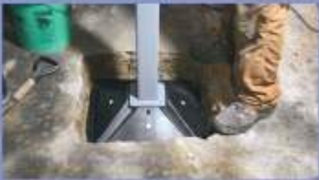
3. Place and secure stabilizer on the LightFoot base.
