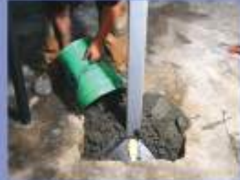
7. Replace and finish concrete when necessary.
